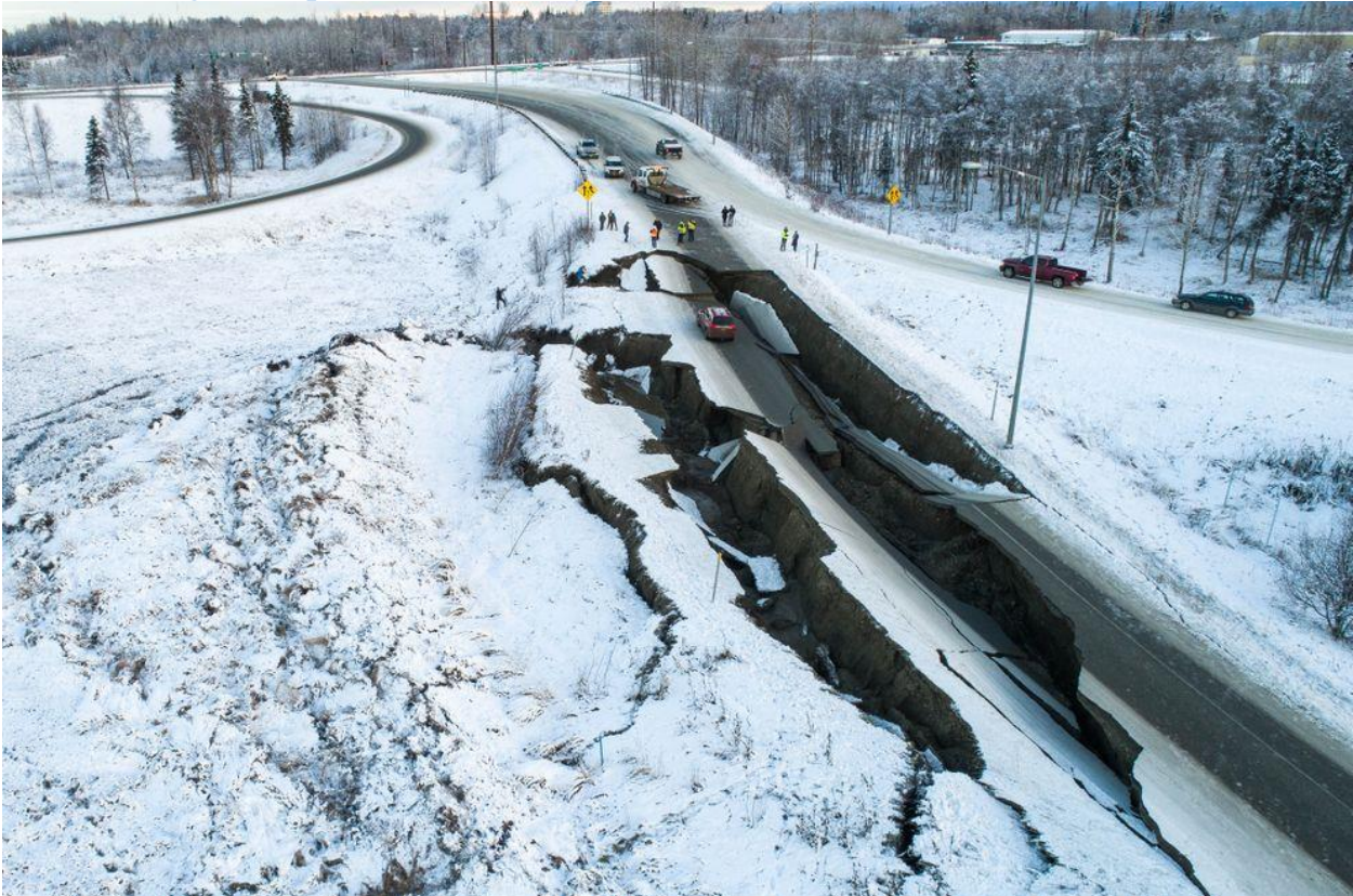
The northbound onramp for International Airport Rd. at Minnesota Blvd. collapsed Friday morning, Nov. 30, 2018 after a strong earthquake shook southcentral Alaska. (Courtesy Ryan Marlow / Alaska Aerial Media)
